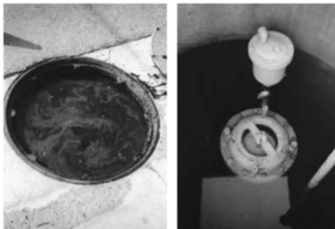
FIGURE 1. Submerged Air Valve Vault (LeChevallier)
