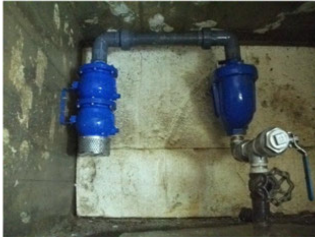
FIGURE 4. Typical ASSE 1063 Inflow Preventer Installation
