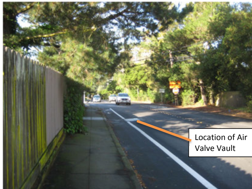
FIGURE 5. Water Pipeline in Foster City, CA
